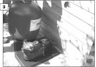
3 Place the filter on the pedestal and fill it with a 1/3rd water.
