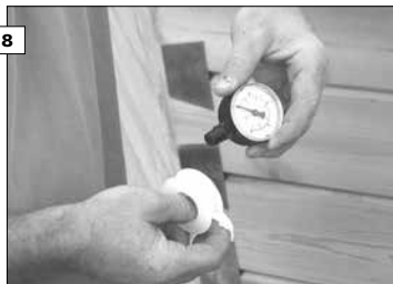
8 Now apply Teflon tape to the outer thread of the manometer.
